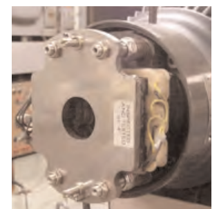
3. Connect wiring and replace cover
